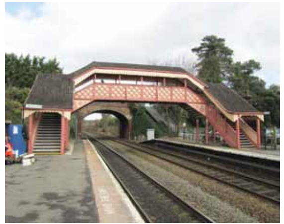
Hagley Station Footbridge
